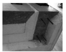
Figure 2: Double L-insulation in ground construction, Värnamo
