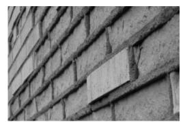
Figure 10: Worn out brick façade, Alingsås
